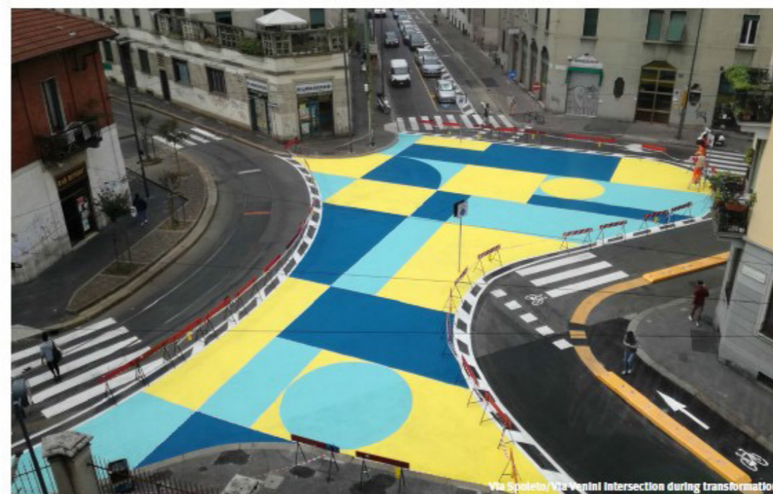
Via Spoleto/Via Venini Intersection during transformation
