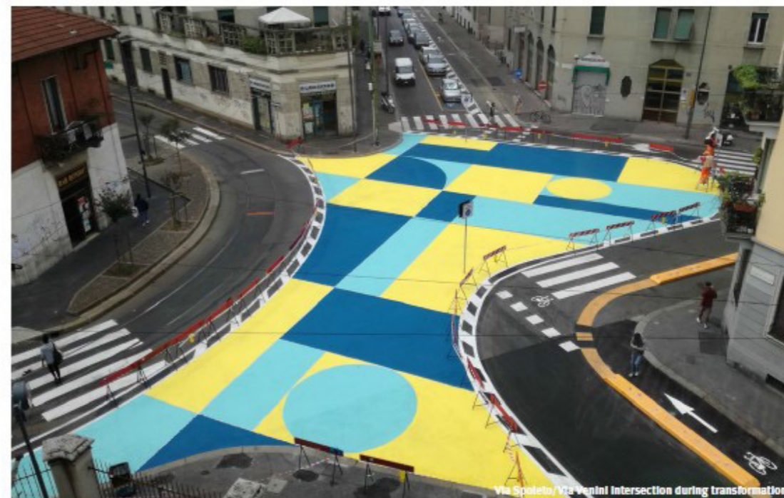
Via Spoleto/Via Venini Intersection during transformation
